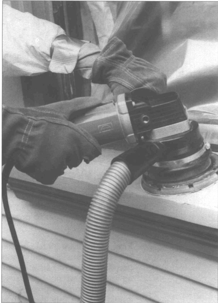
HEPA vacuum-exhausted power sander.
